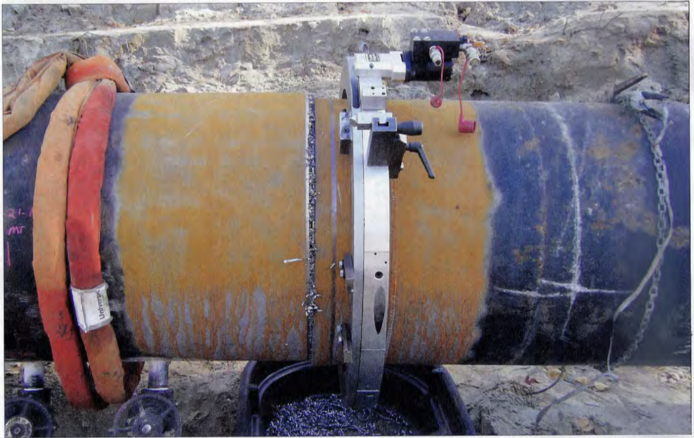
Low clearance split frame shown after making the "money cut." The LCSF is part of a complete machining system ideal for pipeline repair.
