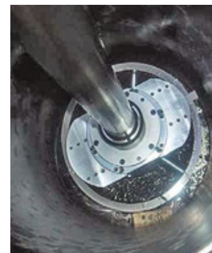
Internal cutting module lowered to cutting depth
