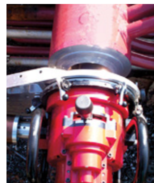
EP 424 AutoFeed deluxe prepping heavy wall pipe
