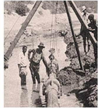
Early pipe fitting
