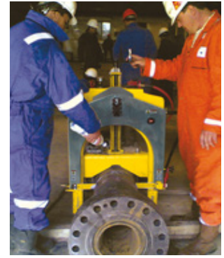
Guillotine cutting pipe
