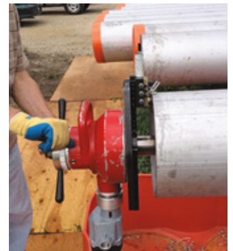
SDB pipe end preparation
