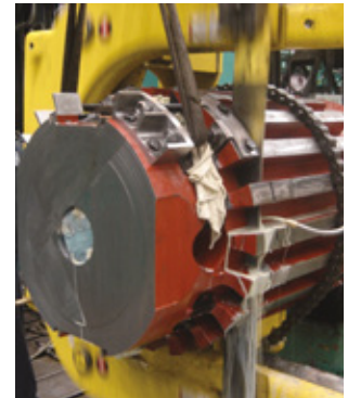
Guillotine Goliath cutting powerplant turbine shaft
