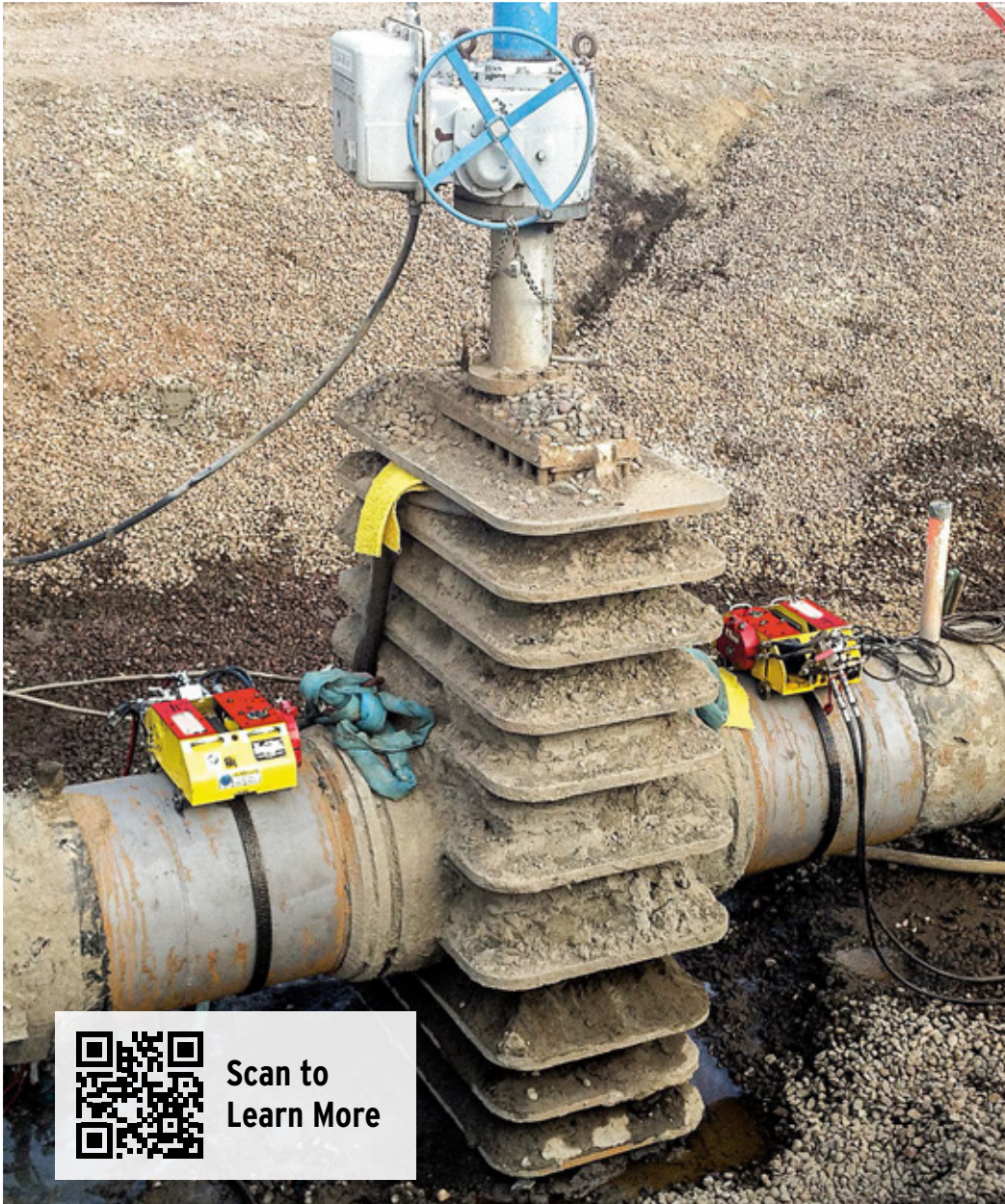
Add mounting chain sections to fit larger diameters
