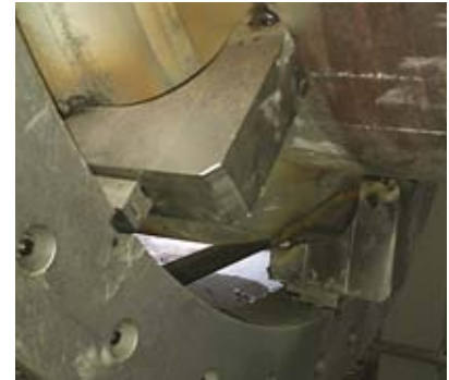
Figure 4 - Custom radiused mounting blocks tacked in place
