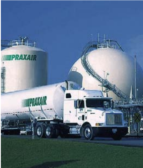
Figure 1 - Praxair is a worldwide provider of industrial gases
