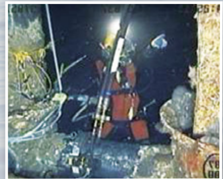
Diver positions split frame prior to cut
