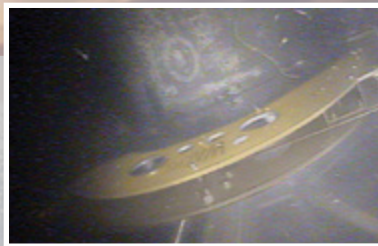
Wachs Diamond Wire Saw in position on a platform leg
