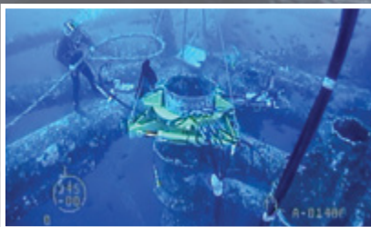
Wachs Dual Pin Drill is ideal for platform removal and decommissioning
