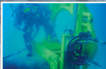
Diver positioning Goliath Subsea Guillotine saw horizontally
