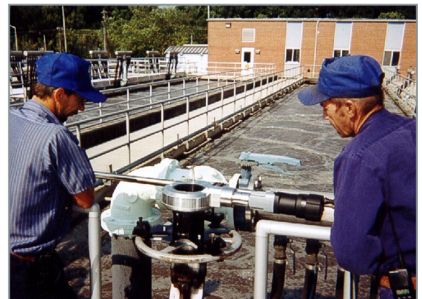
Electric RS-2 available with torque control, shown with handwheel adapter
