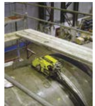
Trav-L-Cutter being used for submarine decommissioning
