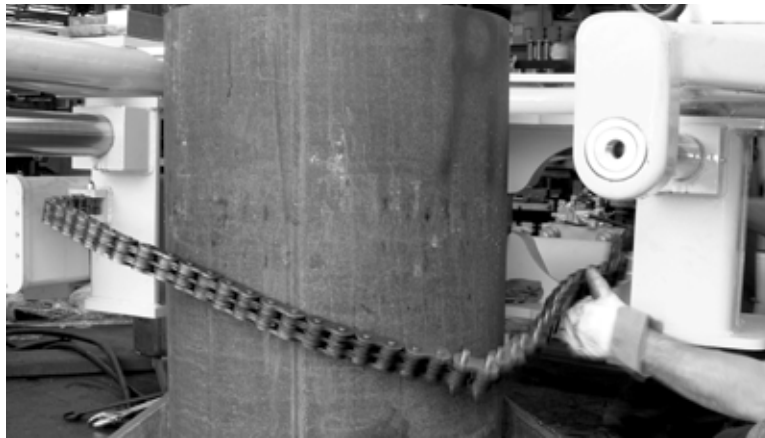
Figure 5-19. With the crane holding the saw in place, wrap the clamping chain around the workpiece.
